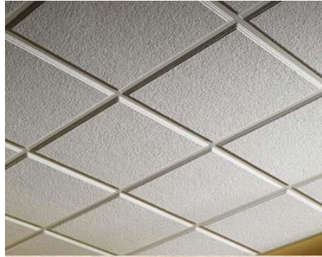
gypsum board false ceiling
