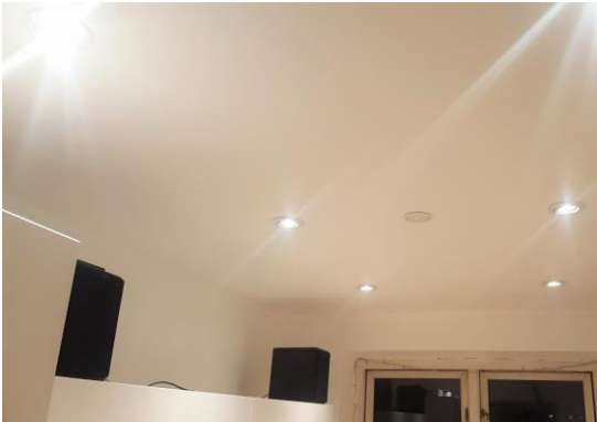
Gypsum board ceiling covered in painted POP
