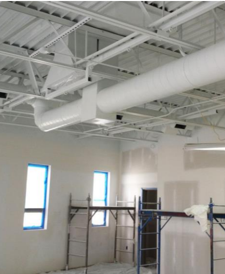
white painted exposed ceiling
