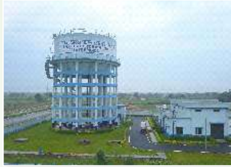
Water Reservoir for 24 x 7 water Supply
