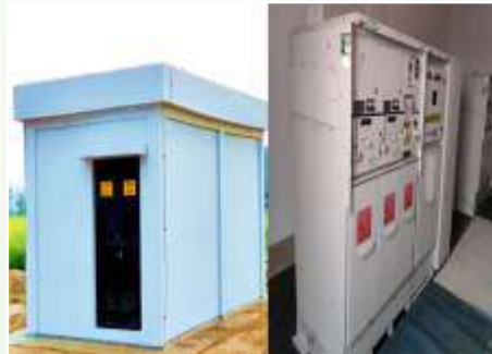
Dedicated RMU Building for each plot for electricity and Optical Fiber Connection
