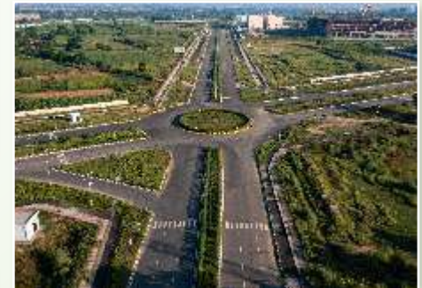
Wide roads with service lane, cycle track and pedestrian path and all utility ducts beneath
